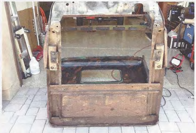
A rotisserie was not available while the pickup was being disassembled, so the underside of the cab—small and lightweight compared to that of other vehicles—was inspected by simply tipping it onto its back. The floor and mounting points were devoid of damage.
